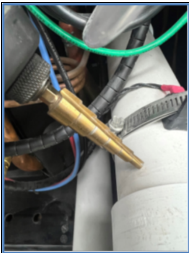
Figure 11- Drill Hole for Sensor
