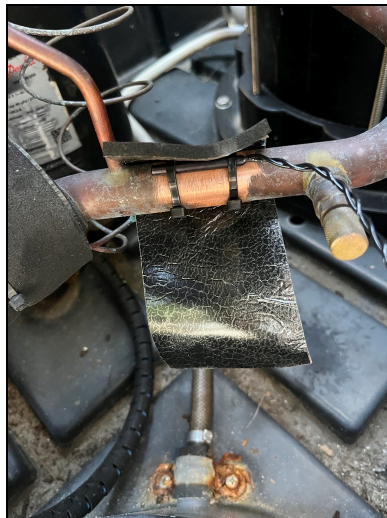
Figure 15- Applying Wrap to Sensor
