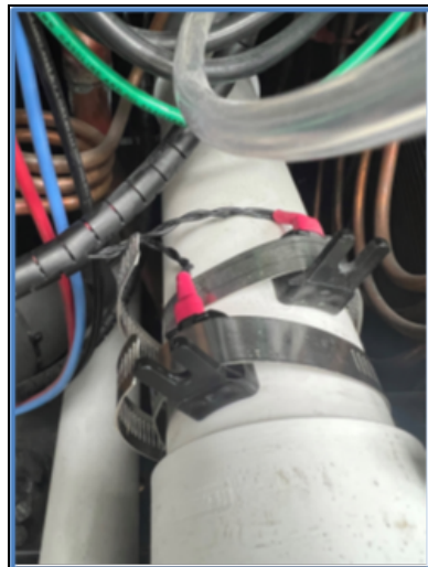
Figure 12- Clamp on Sensor
