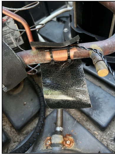
Figure 14- Applying Wrap to Sensor
