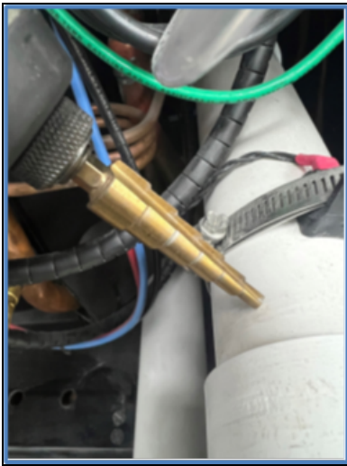
Figure 10- Drill Hole for Sensor
