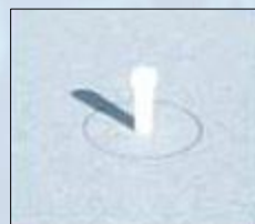
4. Clean hole and insert anchors.
