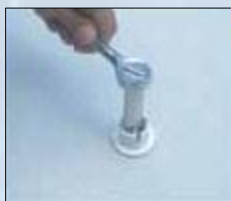
5. Firmly attach mounting caps with provided lag bolts and washes.
